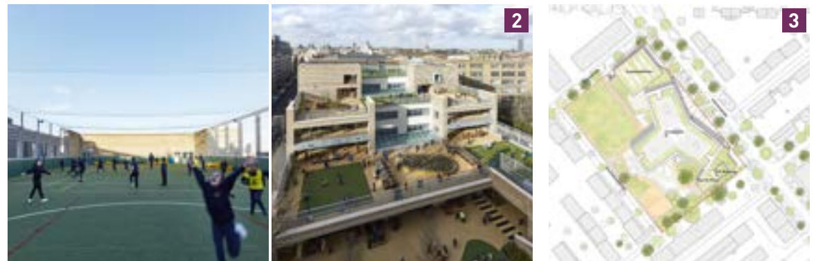
Fig. 186. [2] Marlborough Primary School, Londres, Royaume-Uni; [3] Implantation type, Primary School Infanteriestrasse, Munich, Allemagne. (Sources : Dixonjones, Bernish Arkitekten).
